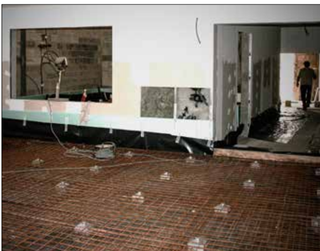
Installation of FZH+Sylomer floor mounts on a recording studio in Spain.
