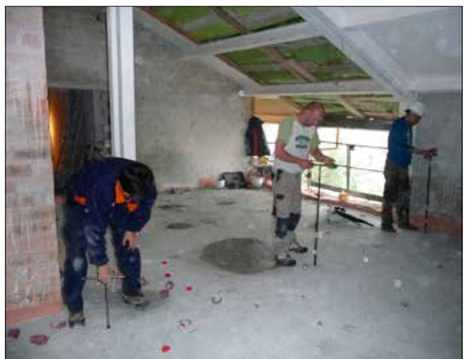
Installation of an FZH+Sylomer ® floor mount.
